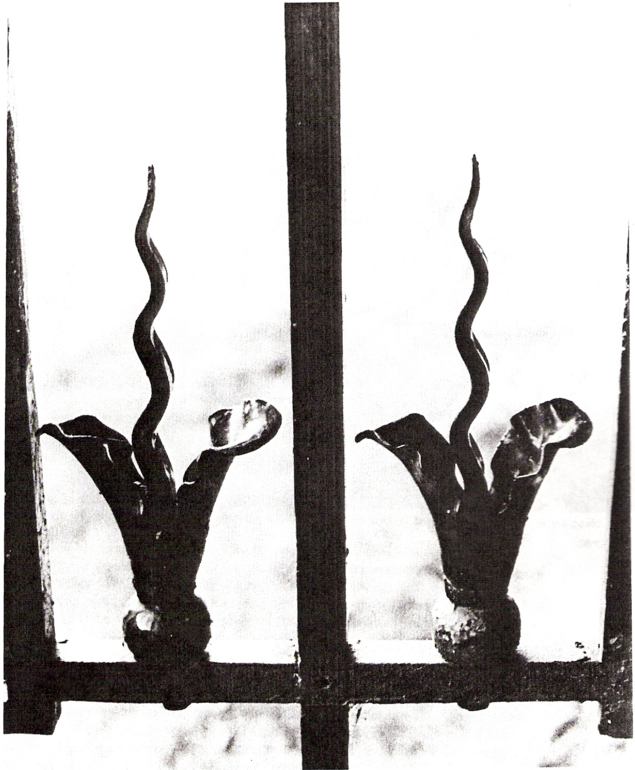
Figure 5 - Sheet Steel is Formed into Leaves around a Drawn-Out Flamelike Centre in each Decoration
