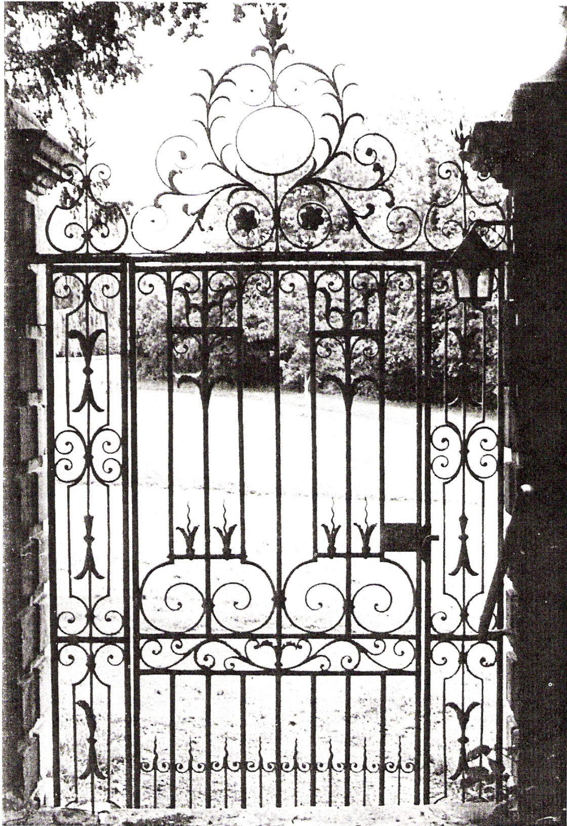
Figure 4 - This Church Gate Shows How Scrolls and Leaves can be Built up into a Very Effective Whole Design
