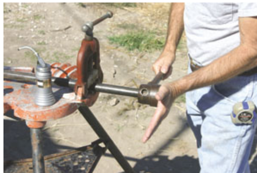
Threading the end of a pipe
