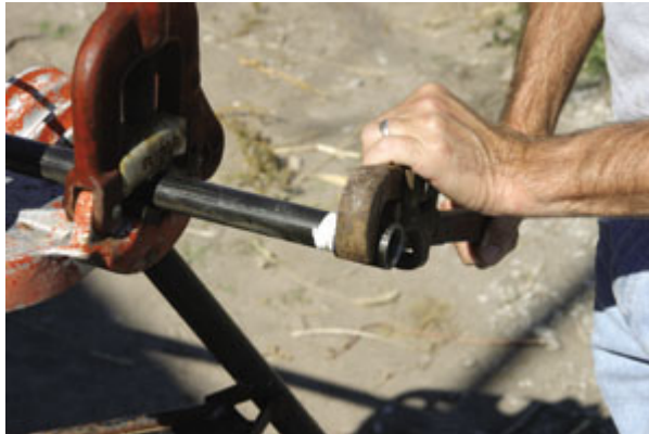
Tighten the coupling or fitting by turning one and a half more turns after hand tight
