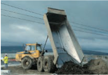
Figure 12–Hazard from overhead cables and the method employed to eliminate the risk
