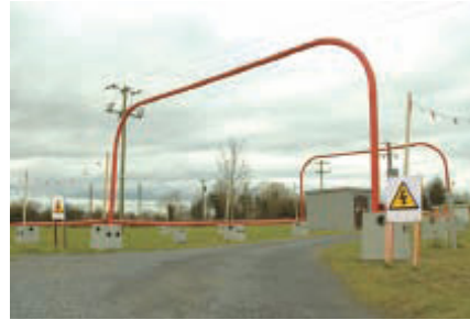
Figure 12–Hazard from overhead cables and the method employed to eliminate the risk
