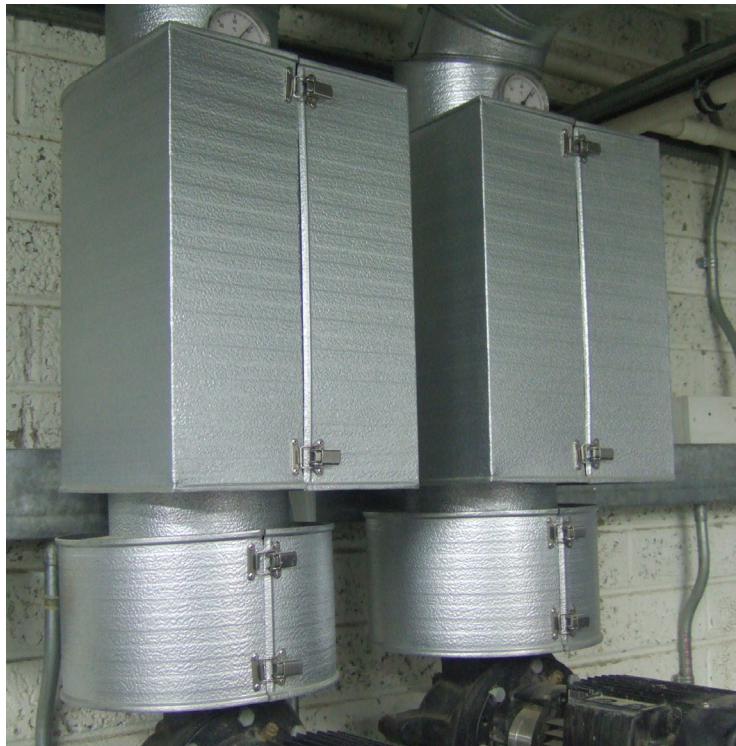
Valve and Flange Box Arrangement.
