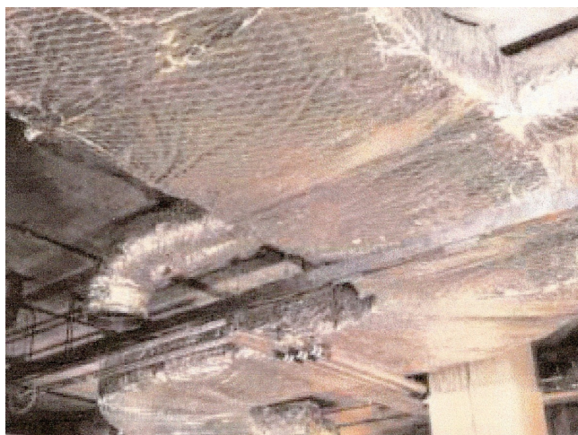
Rockwool duct wrap used to thermally and acoustically insulate ducting.
