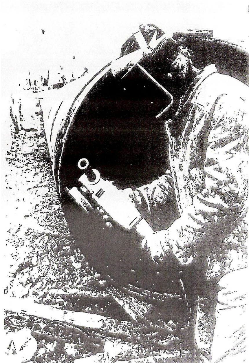
Figure 6 – (b) Angle Grinder used for Bevel Grinding
